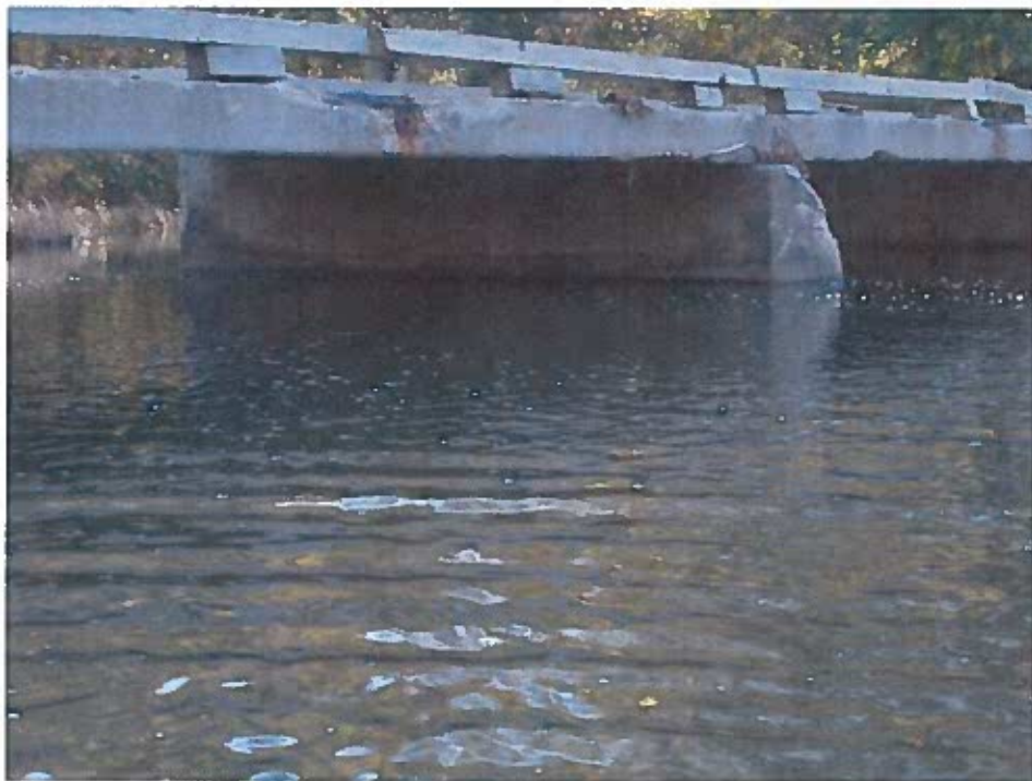
Pier 3 Elevation – Looking Northeast and Lateral Tensioning Rods Spans 2 & 3
