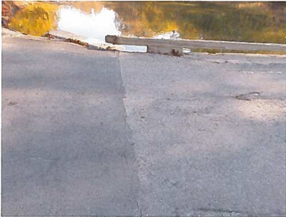
Abutment 1 Joint
