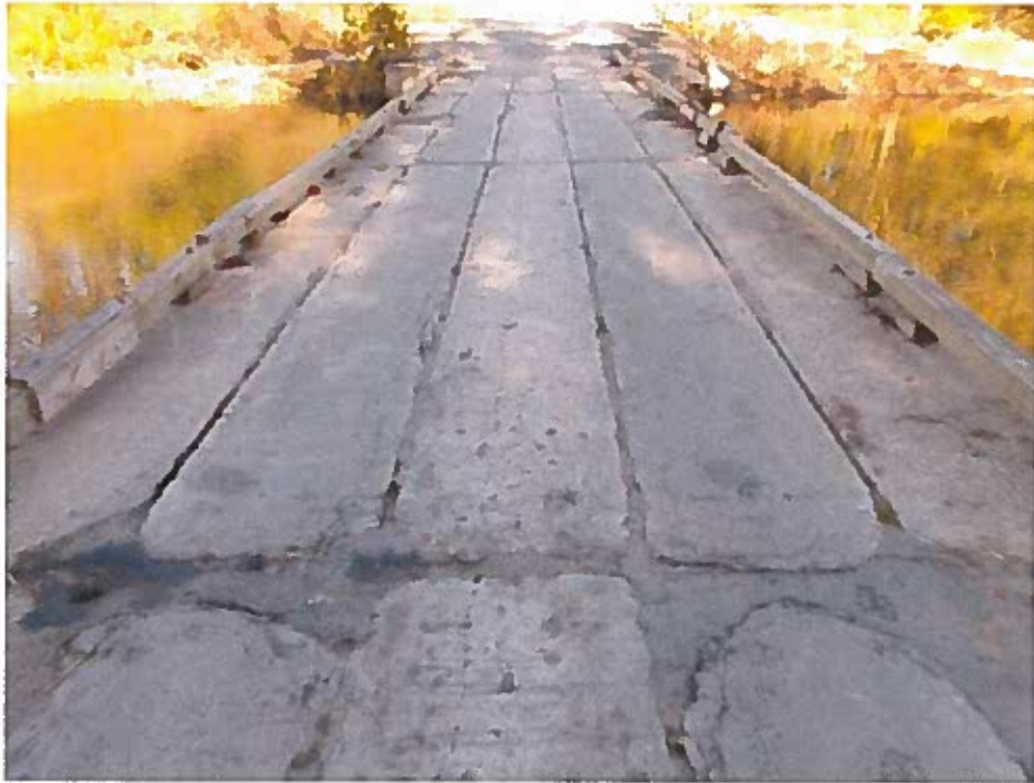
Bare Concrete Deck, R/Conc Box Girders, and Longitudinal Shear Keys (Typical)
