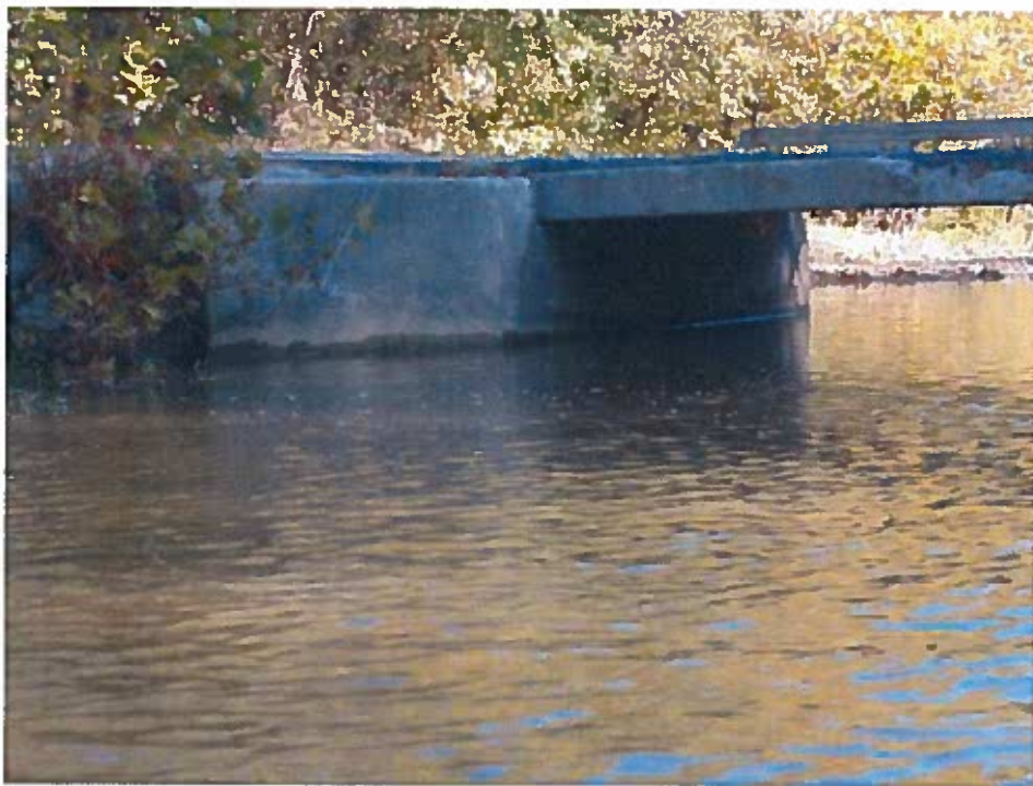
Abutment 1 Elevation – Looking Northwest
