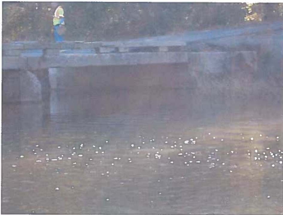
Abutment 5 Elevation - Looking Northeast
