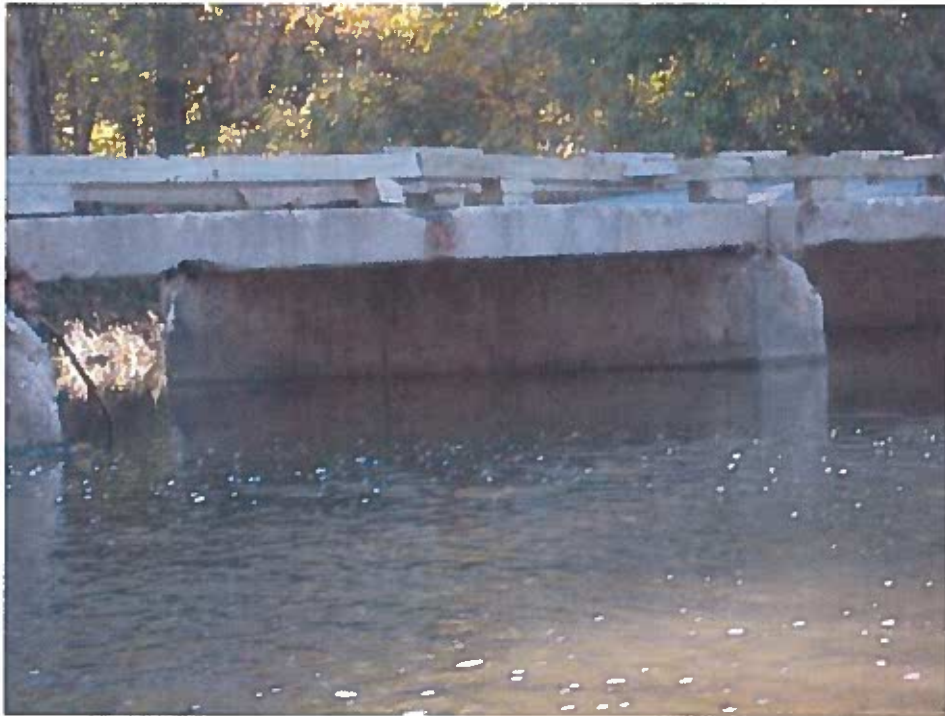
Pier 4 Elevation – Looking Northeast
